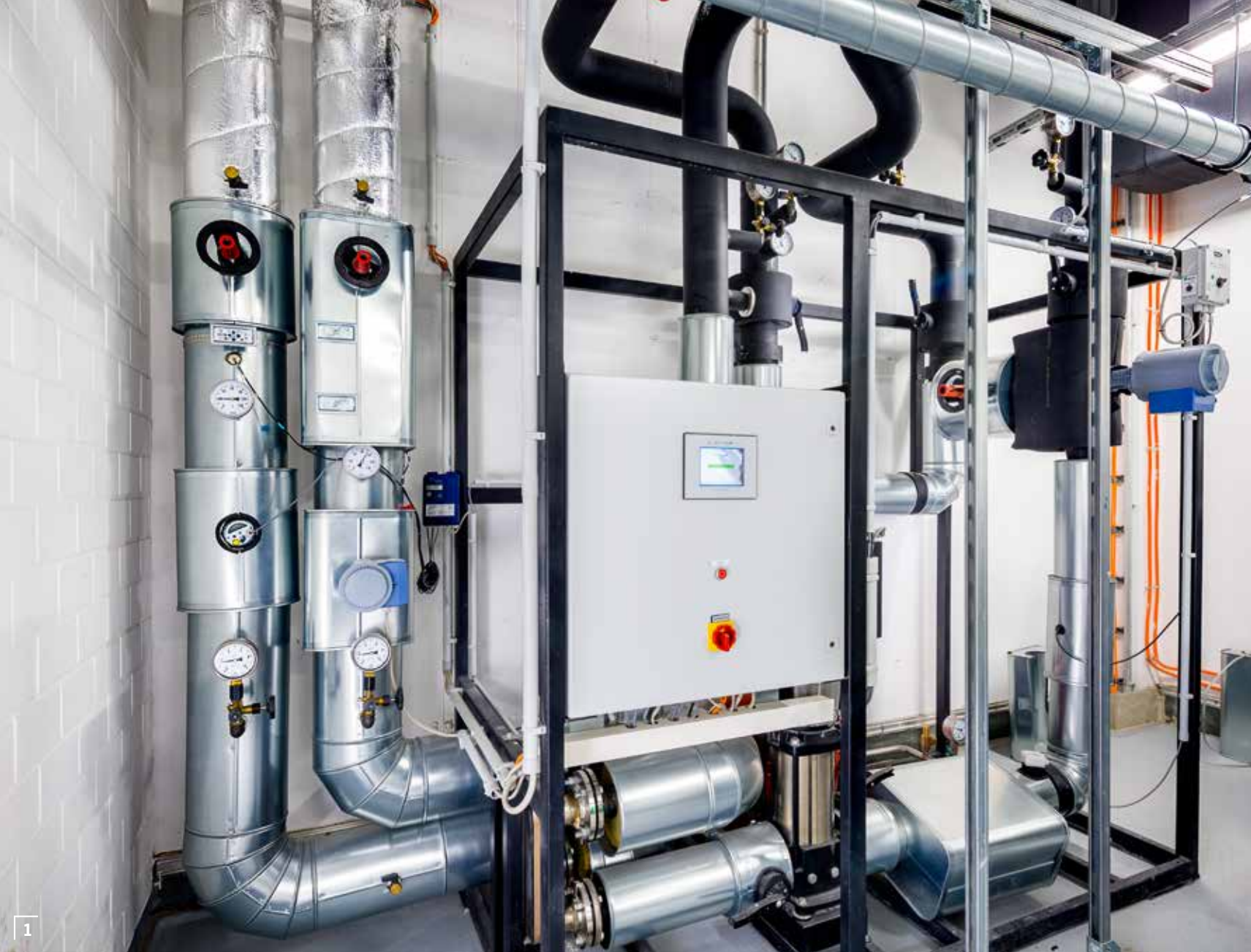
1 // Highly efficient heat recovery system EcoCond as a circulation system with integrated heat refeeding 2 + 3 // Central air conditioning unit for office air conditioning with high-performance circulation system EcoCond
